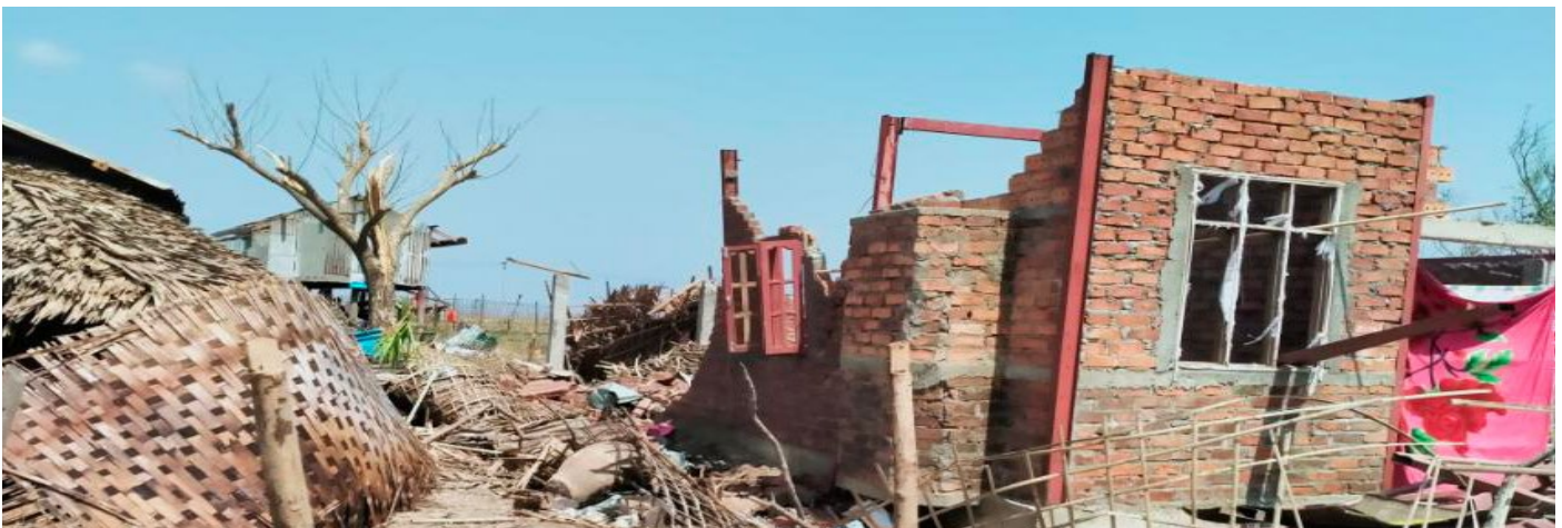
Destroyed brick and bamboo houses in Rathedaung township. Photo: IOM Myanmar
